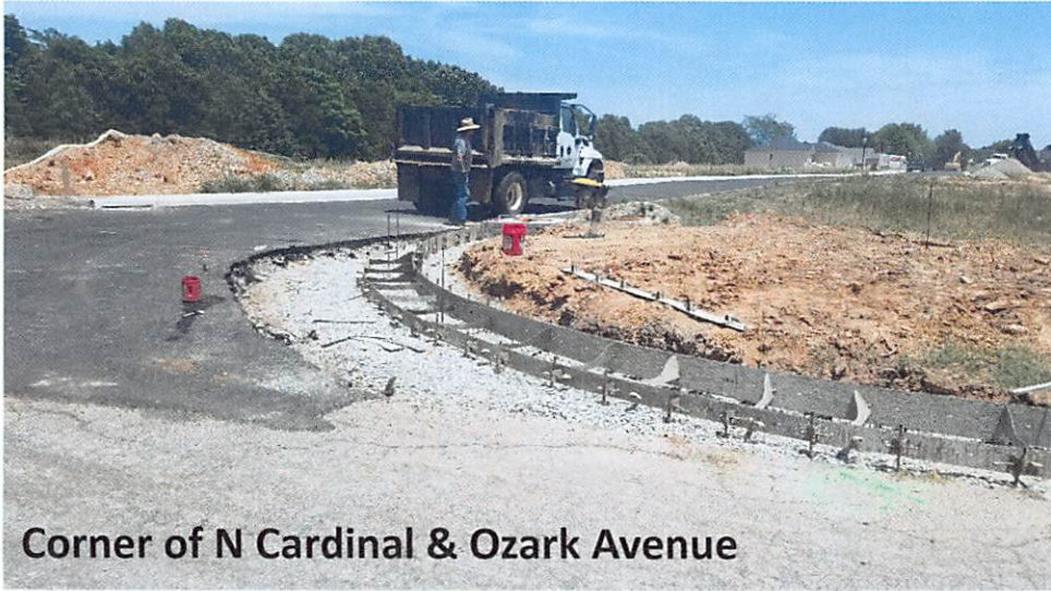
Curbs at easement to connect both sides of Ozark Avenue
